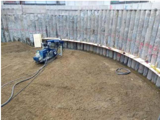
DPT dengan countinues pile (borpile).
